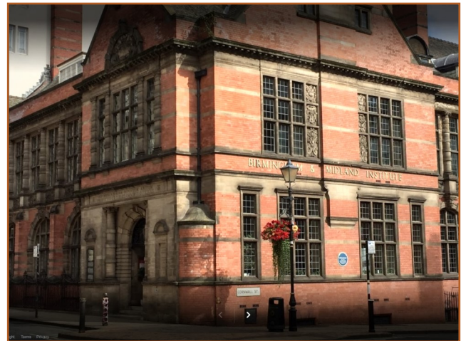
Figure 5: Birmingham and Midland Institute (courtesy https://www.google.com/maps/ ).
